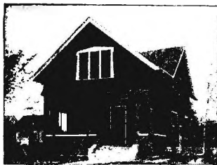
A No. 2-19-W IDEAL Boiler and 340 sq. ft. of 38-in. AMERICAN Radiators, costing owner $166, were used to heat this cottage. At this price the goods can be bought of any reputable, competent Fitter. This did not include cost of labor, pipe, valves, freight, etc., which are extra, and vary according to climatic and other conditions.
